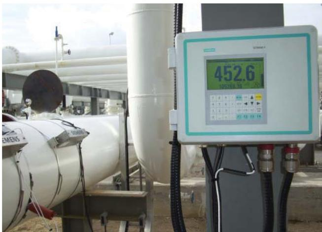
Typical clamp-on Ultrasonic Flowmeter installation on hydrocarbon pipeline
