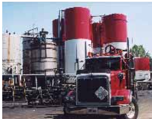
A new ultrasonic level monitoring system at the PSC Philip Services plant in Rexdale provides reliable data that allows for effective scheduling and accurate inventory control.
