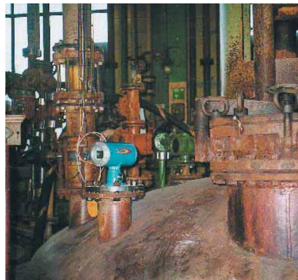
DyStar Textilfarben GmbH & Co. in Leverkusen, Germany, uses the SITRANS LR 300 for reliable level measurement of pigment
