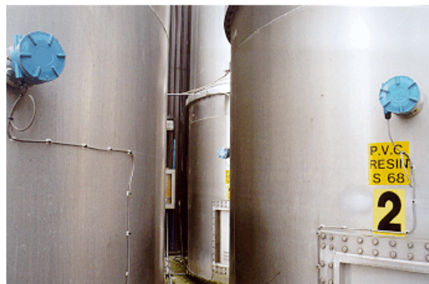
Milltronics Mercap measures dusty PVC powder levels to ensure maximum production efficiency at Anglian Windows.
