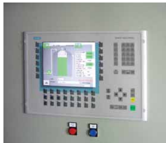
The Siemens HMI provides the status of each tank with visual cues indicating level.
