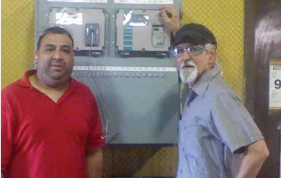
Siemens Level Specialist Al Dhanji worked closely with Ron Odom, Electrical Engineer, Georgia Pipe to provide the best level measurement solution for plastic resin and reclaimed plastics – two Sitrans LU10 and sixteen Echomax XPS-30s.
