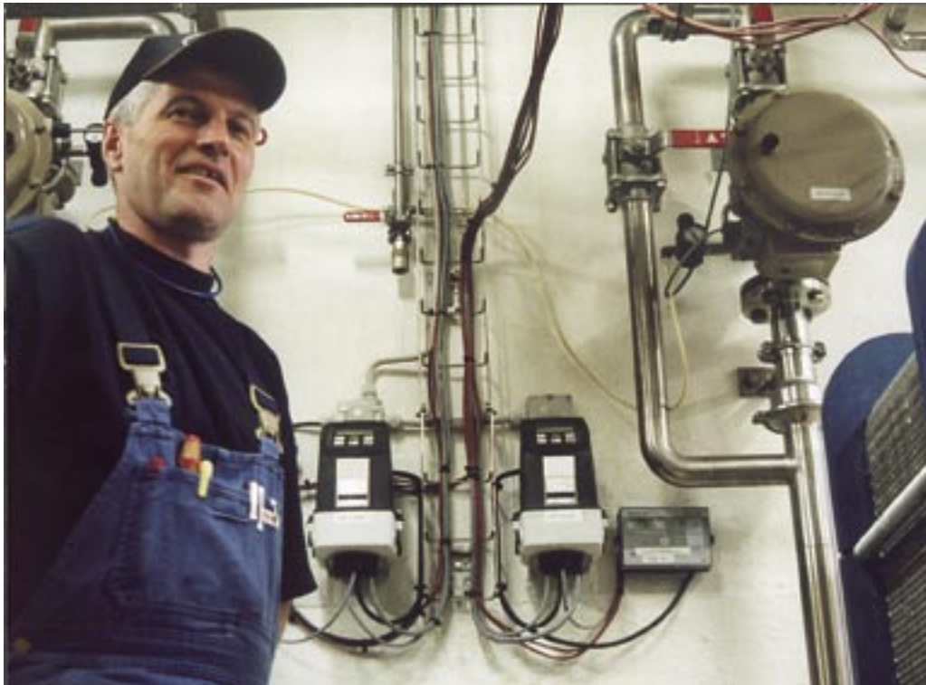
Allan Petersen standing next to two of the Arla Food Samden flowmeters for custody transfer: "There is much money involved even if the inaccuracies are minor".
