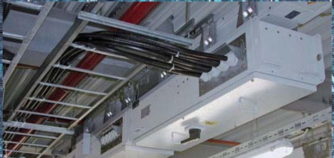
3VL circuit breakers protect tap-off units up to 1,250A. An LD busbar trunking system enables hot swapping
