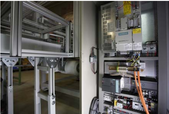
Integration from one source: Besides the sensors, the remaining controller technology and the drives also come from the Simatic product range by Siemens
